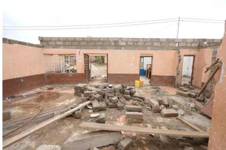
Kombayendeh Community Health Centre during PIH renovation
