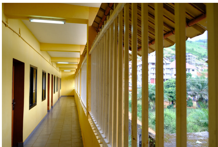
The MDR-TB ward, last year amid construction. Patient rooms are on the right.
